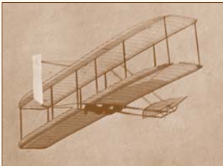
The 1902 Glider with three-axis control system in a coordinated turn
